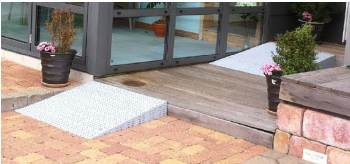
Type I ramps with the inclination angle of 14,5%.
