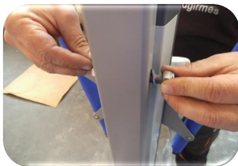
Picture 5: Now attach the locking nut.
