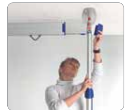
Fix end cap to lock rail in place.
